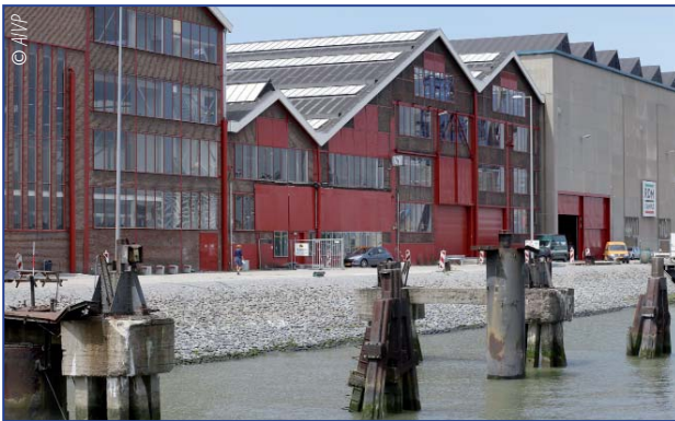
Rotterdam - RDM Campus: education and technological innovation site
