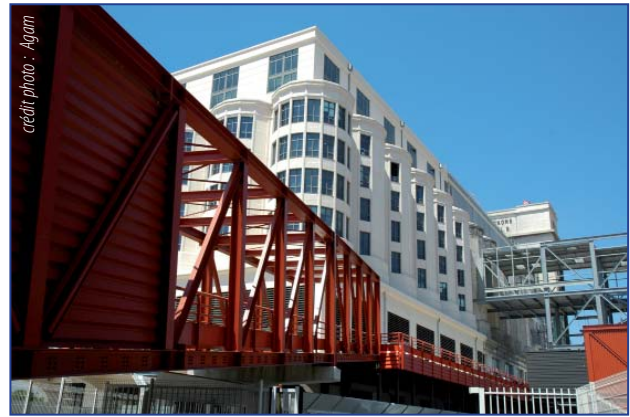
Marseille - Conversion of a former silo into a concert hall
