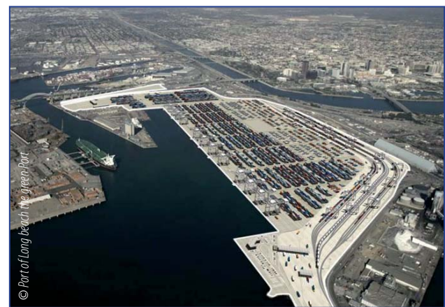
Long Beach - Recomposition project: Middle Harbor Redevelopment
