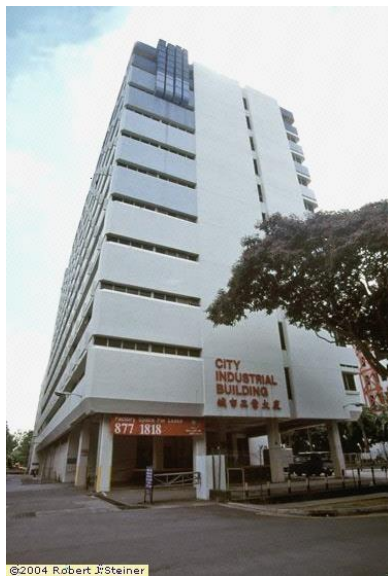
City Industrial Building
